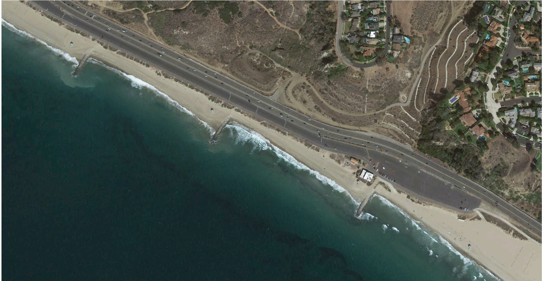
Groins along Pacific Coast Highway, in Pacific Palisades, Los Angeles, California
